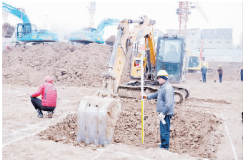
挖下柱墩基槽
